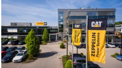
The Zeppelin Power Systems site in Achim:
